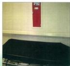
Fire alarm pull station, extinguishers, and medial gas shutoff valves should **NEVER** be blocked!
